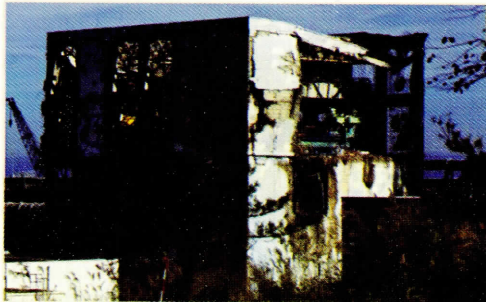
Fukushima Daiichi Power Plant damaged by earthquake and
