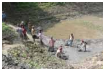
Plate 17: Clayey soil were being dug from the base of ditch to maintain homestead floor. (in 2007.3)
