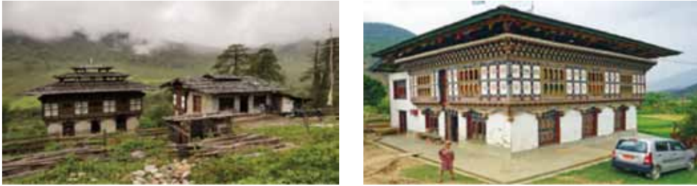
Figure4: Houses before (left) and current (Right)
