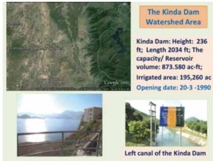
Photo4: Kinda dam (Khin and Ando 2015)
