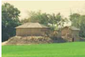
Plate 15: Started to live one month after the construction. Bananas are growing. (in 1993.3)
