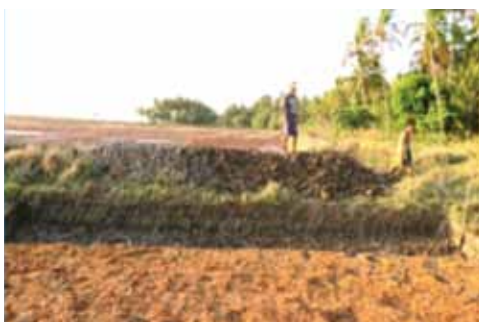
Photo2: Embankments in Auk Seik Kwin village
