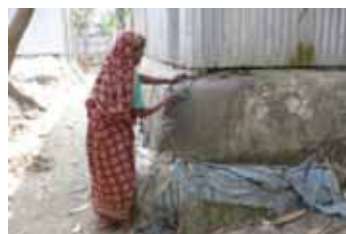
Plate 19: Base of building is maintained regularly with care by women. (in 2007.3)
