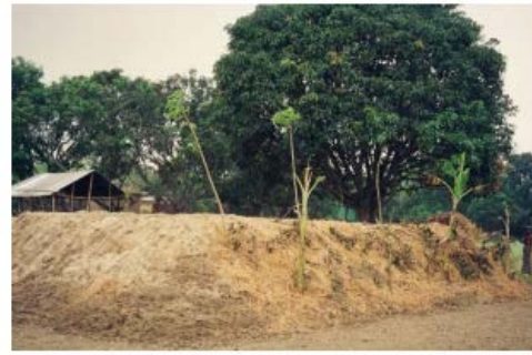
Photo 3.3 Planting vegetation on the periphery of raised mound
