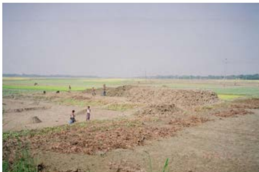
Photo 3.1 Digging of soil for raised mound
